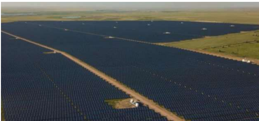
On photo: 100MW Saran Solar Park (financed by EBRD and GCF)
